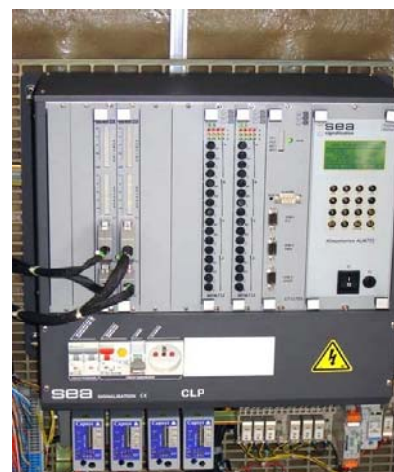
IVR connected to the traffic lights controller
