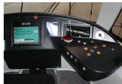
Track-switching command panel
